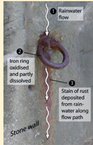
An old iron ring in a stone wall illustrates the essential elements of rock–water interaction: (1) a water flow path: rainwater running over the stone surface, (2) a site of mineral dissolution: iron ring, (3) a downstream site of mineral redeposition: rusty stain.
